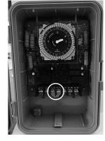
Align the ICM550 so it slides UP and INTO the plastic channels (A), while ensuring the screw holes on the ICM550 line up with the plastic standoffs (B) on the enclosure
